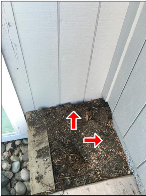
2.4 Item 1(Picture) planter box burring siding
