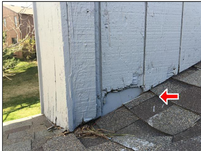
2.4 Item 4(Picture) back side of chimney
